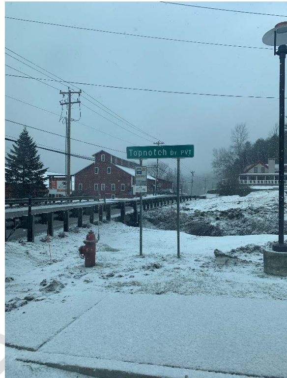
Figure 42: Sight Distance Challenges Exiting Top Notch Resort
