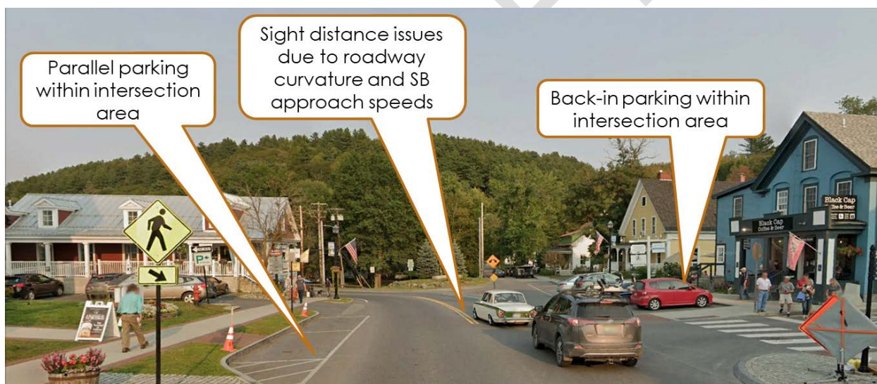
Figure 35: VT 100/School Street/Sunset Street Intersection (Image: Google Streetview)
