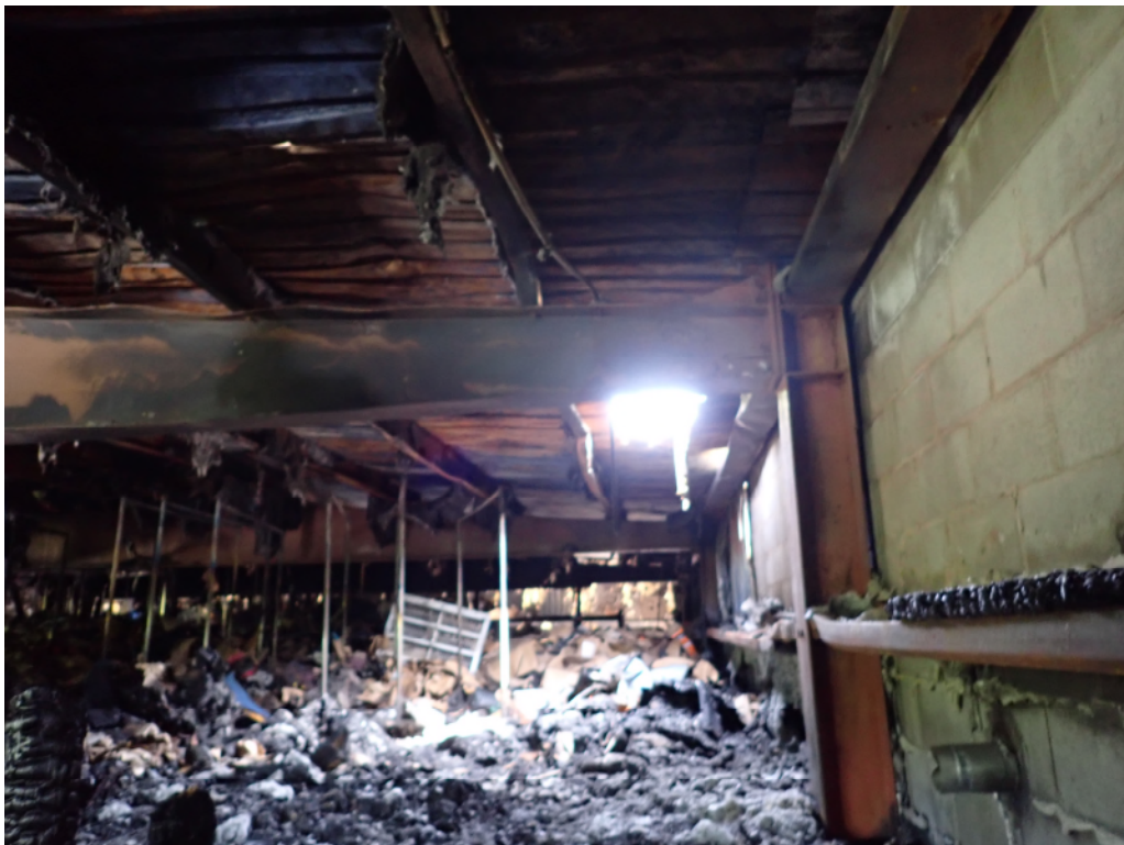
Photo No. 6: The steel framing had been warped by the heat from the fire.
