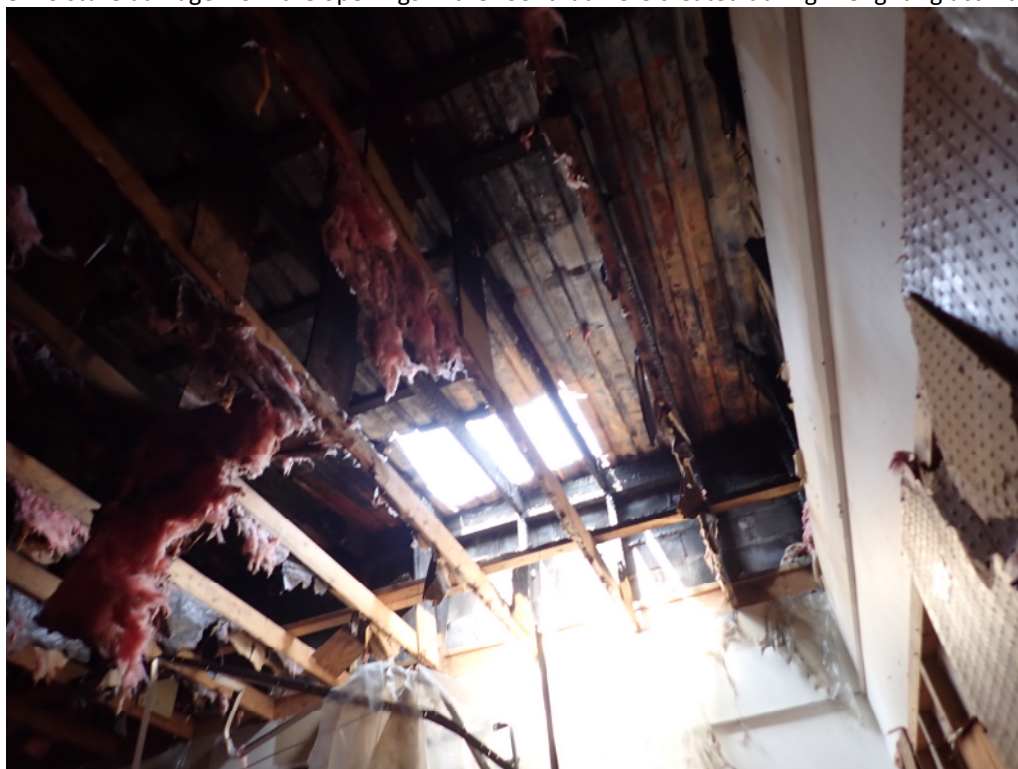
Photo No. 8: Charred wood roof framing, moisture damage below hole in the roof that was created during firefighting activity.
