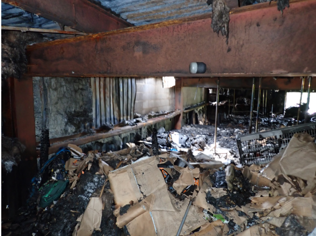
Photo No. 4: The steel framing had been warped by the heat from the fire.
