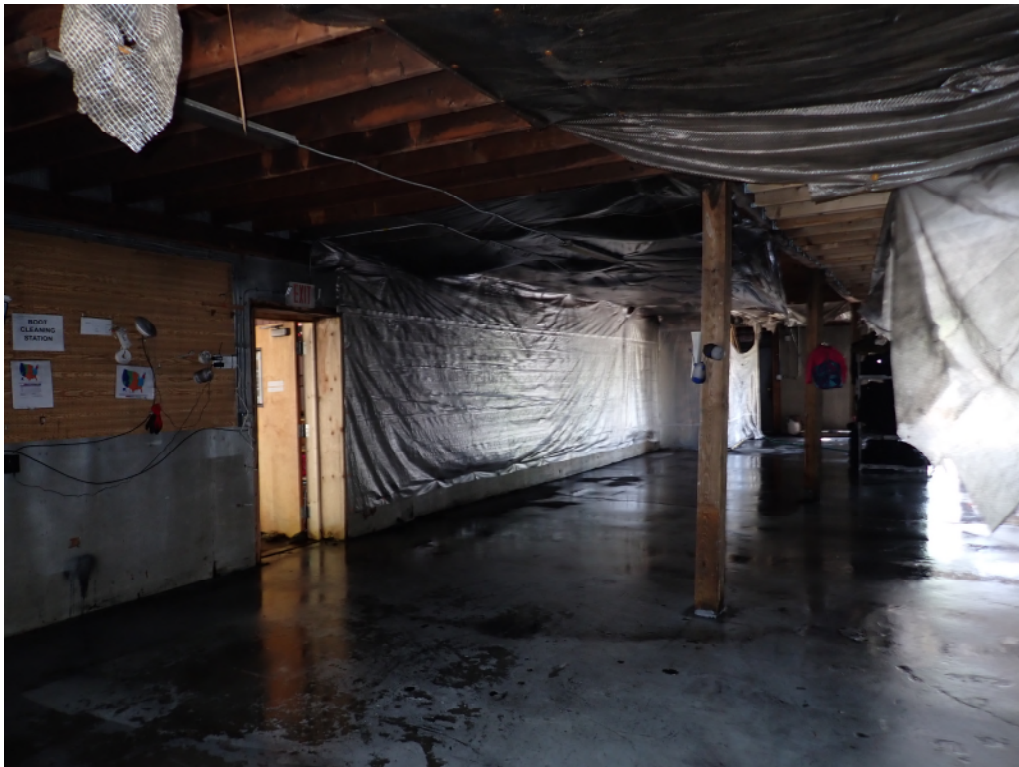
Photo No. 10: Moisture damage below holes in the roof that were created during firefighting activity.
