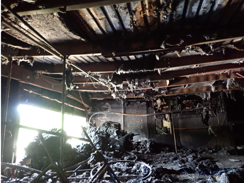
Photo No. 2: Steel framed second story of the subject building. The steel framing had been warped by the heat from the fire.
