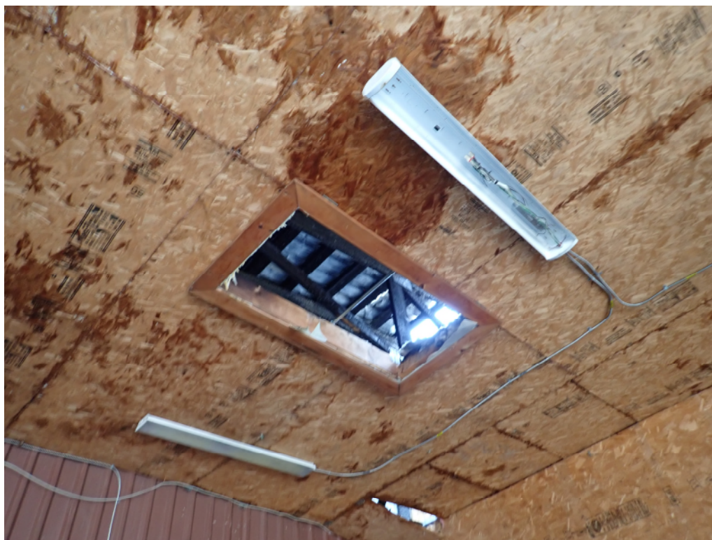
Photo No. 7: Charred wood roof framing above the wood framed east area of the building. There was extensive moisture damage from the openings in the roof that were created during firefighting activity.
