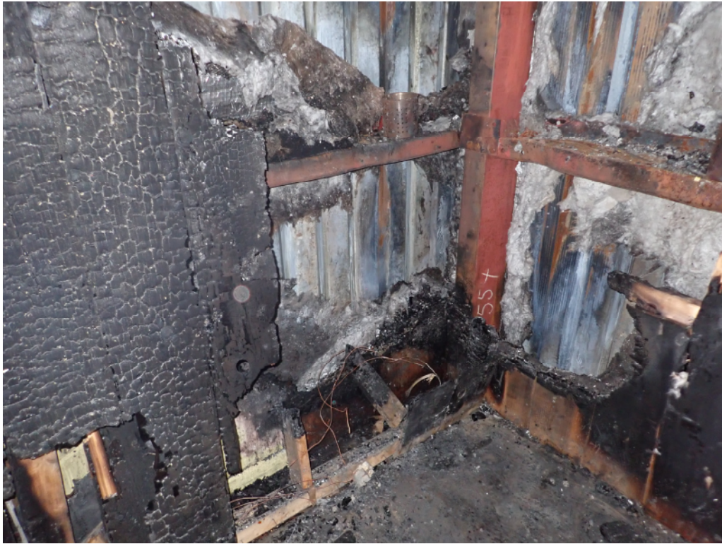
Photo No. 5: The steel framing had been warped by the heat from the fire.
