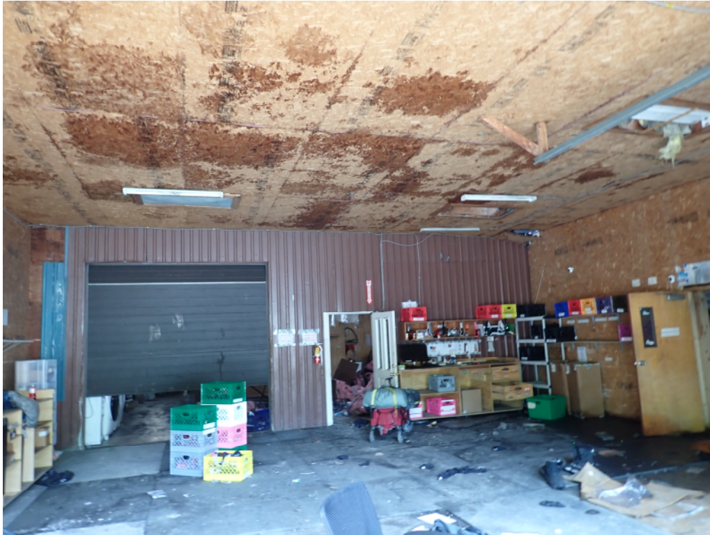
Photo No. 9: Moisture damage below hole in the roof that was created during firefighting activity.
