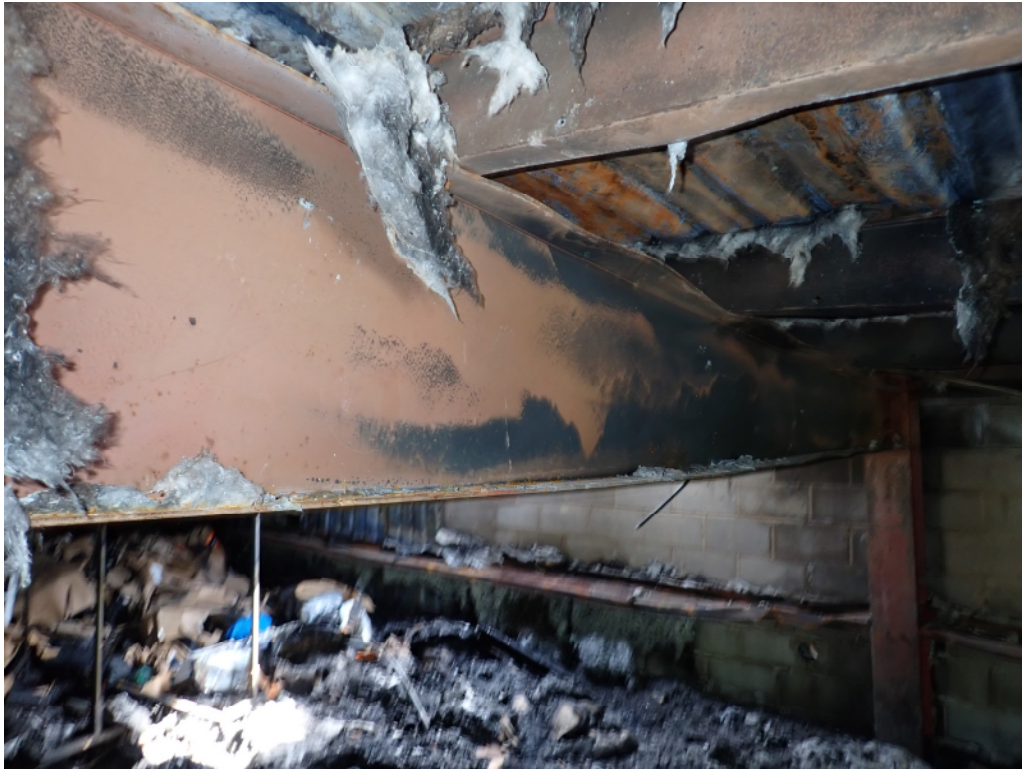
Photo No. 3: The steel framing had been warped by the heat from the fire.
