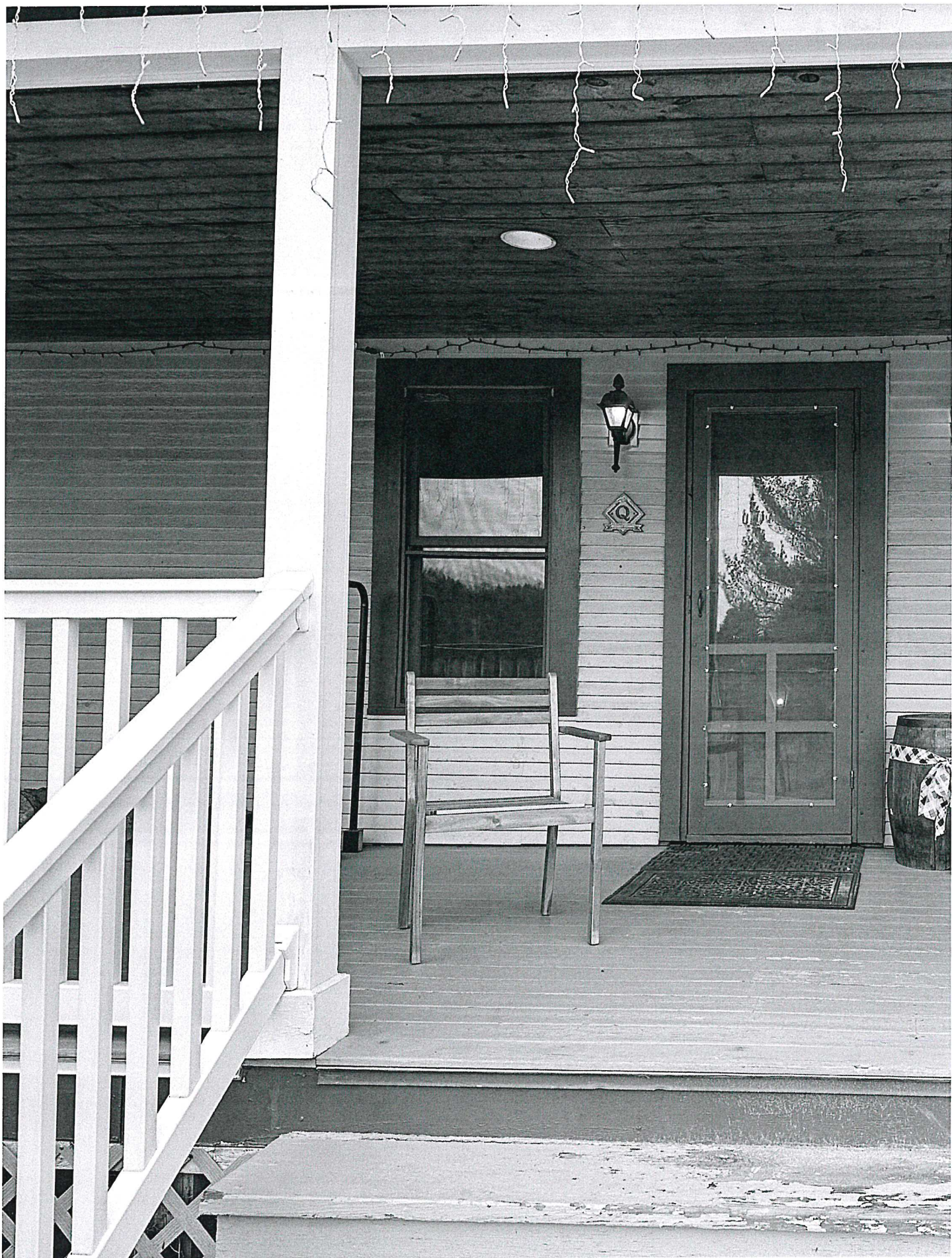
1 Porch on side of house facing driveway
