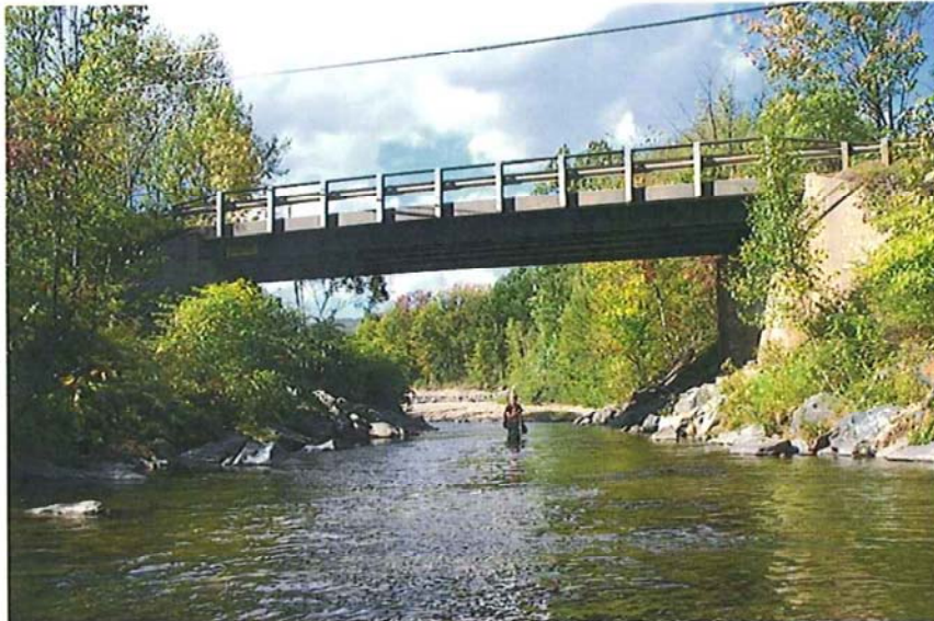
Figure 4. Luce Hill Bridge
