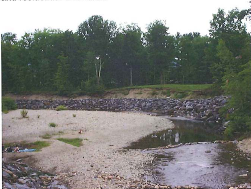
Figure 12. Sediment upstream of Luce Hill Bridge
