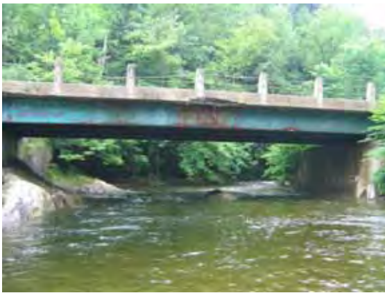
Figure 7.40. Bridge crossing of Nebraska Valley Road constricting Reach T4.02
