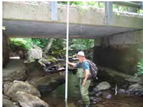
Figure 7.47. Constricting bridge at Nebraska Valley Road in Reach T4.05
