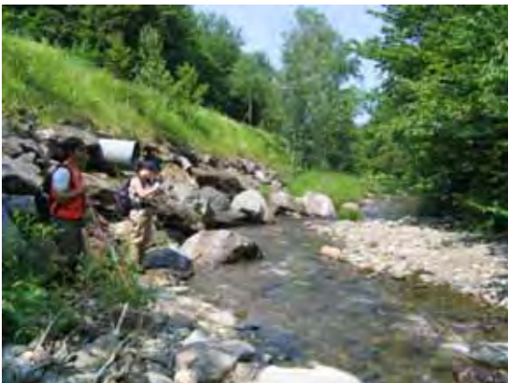
Figure 7.52. Rip-rap armoring, lack of buffer, and stormwater input in Segment T6.03-B
