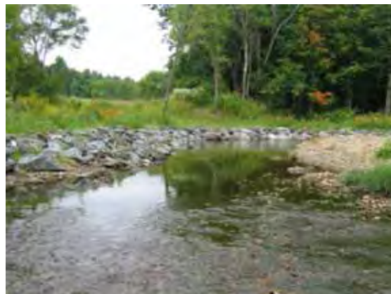
Figure 7.33. Rip-rap along bank upstream of Tansy Hill Road Bridge in M19-B
