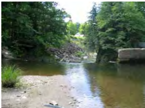
Figure 7.21. Old dam grade control is constricting channel and causing sediment deposition upstream in M15-A.
