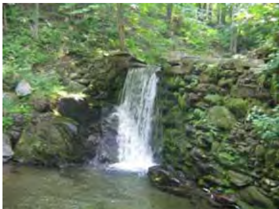
Figure 7.60. Old rock dam grade control in T6.07
