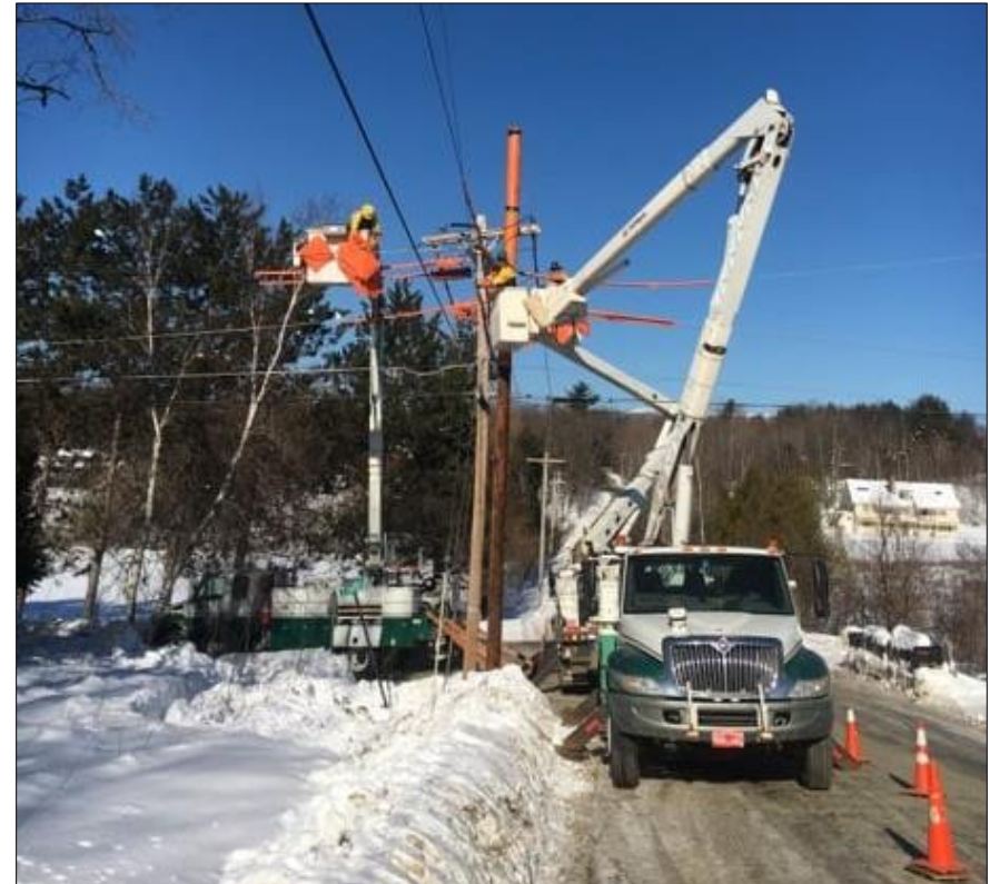
SED line work. Photo credit: Stowe Electric Dept.
