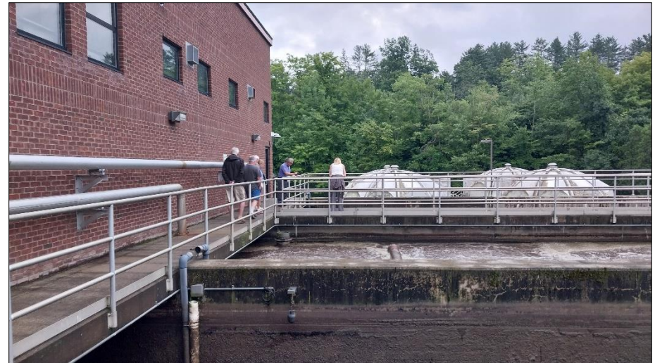
Stowe Wastewater Treatment Facility. Photo credit: Town of Stowe
