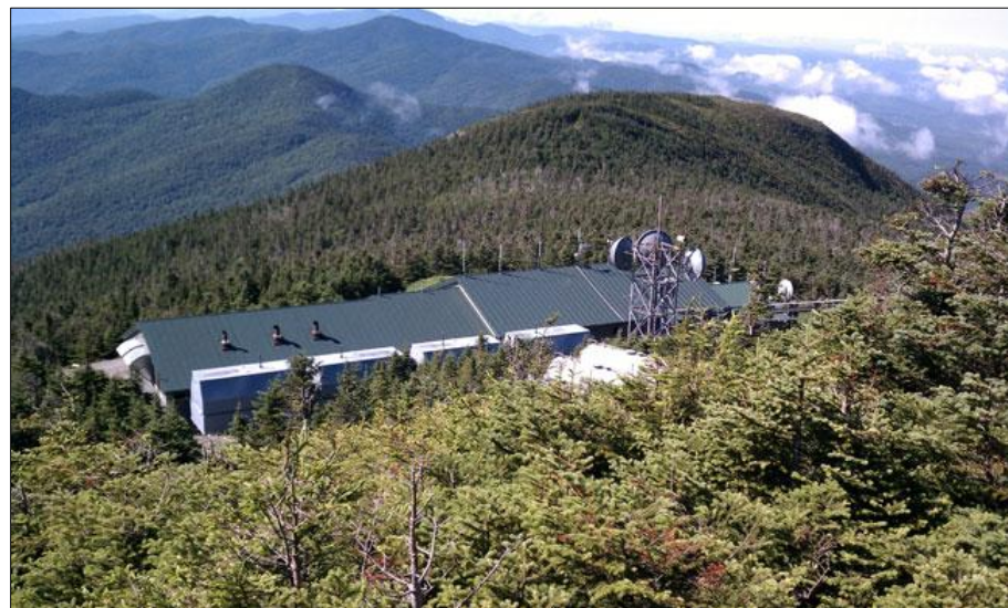
Communication facilities on Mount Mansfield. Photo credit: Town of Stowe
