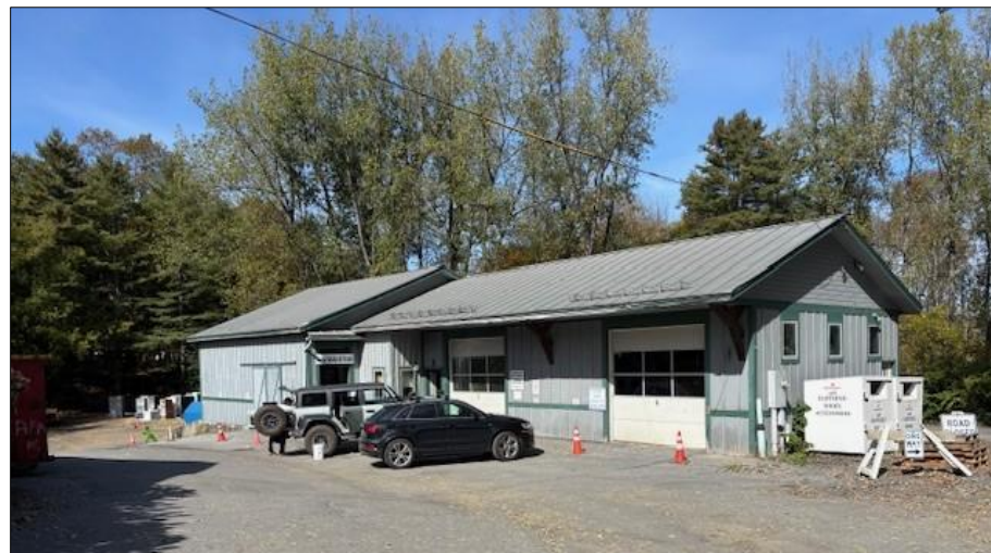
Transfer station on Dump Road. Photo credit: LRSWMD
