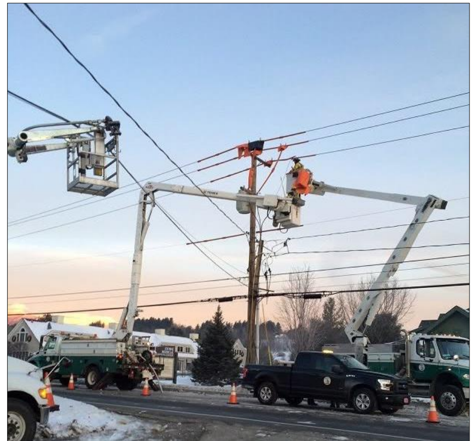
Stowe electric line work. Photo credit: Stowe Electric Department
