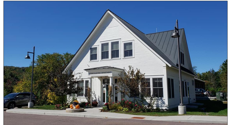
Stowe Electric Office in Moscow. Photo credit: Stowe Electric Dept.
