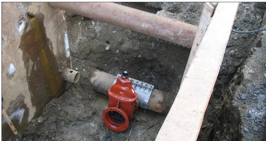
Underground municipal water infrastructure work. Photo credit: Town of Stowe
