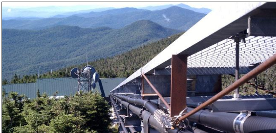
Communication facilities on Mount Mansfield. Photo credit: Town of Stowe
